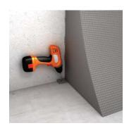
2 Fasten the shower column to the floor by using screws.
