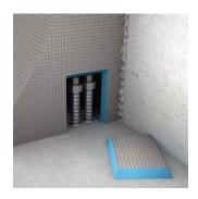
4 Connect cold and warm water supply lines (½) to the units connector threads via the inspection opening at side bottom. Make sure you align wedi connectors and supply pipes before adhesives have set. Test waterproof assembly.
