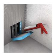
5 Close the inspection opening by applying wedi joint sealant on all four sides of the mitered panel that closes the opening. Seal all seams topically with another bead of wedi joint sealant and spread flat.
